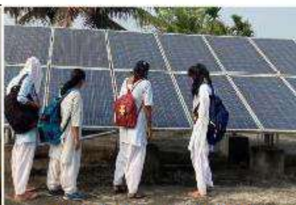
Figure: Rooftop Solar Plants
